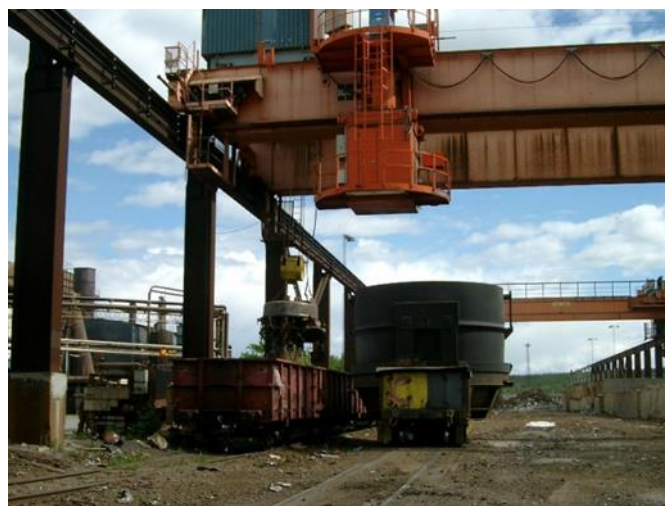
Figure 7: Example of scrap yard with movable rail-bounded scrap bucket
