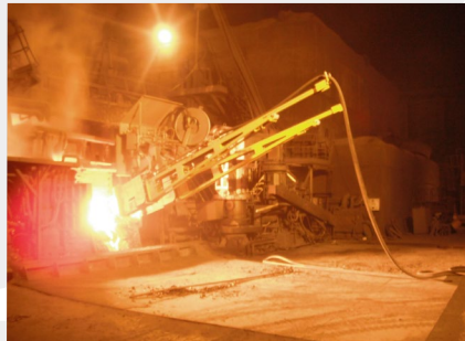
... but the efficiency, reliability and flexibility of the LM.2 convinced the floor personnel and executives straightaway.
